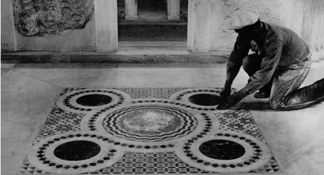
50. Laying the Floor Panel under the Dome.
