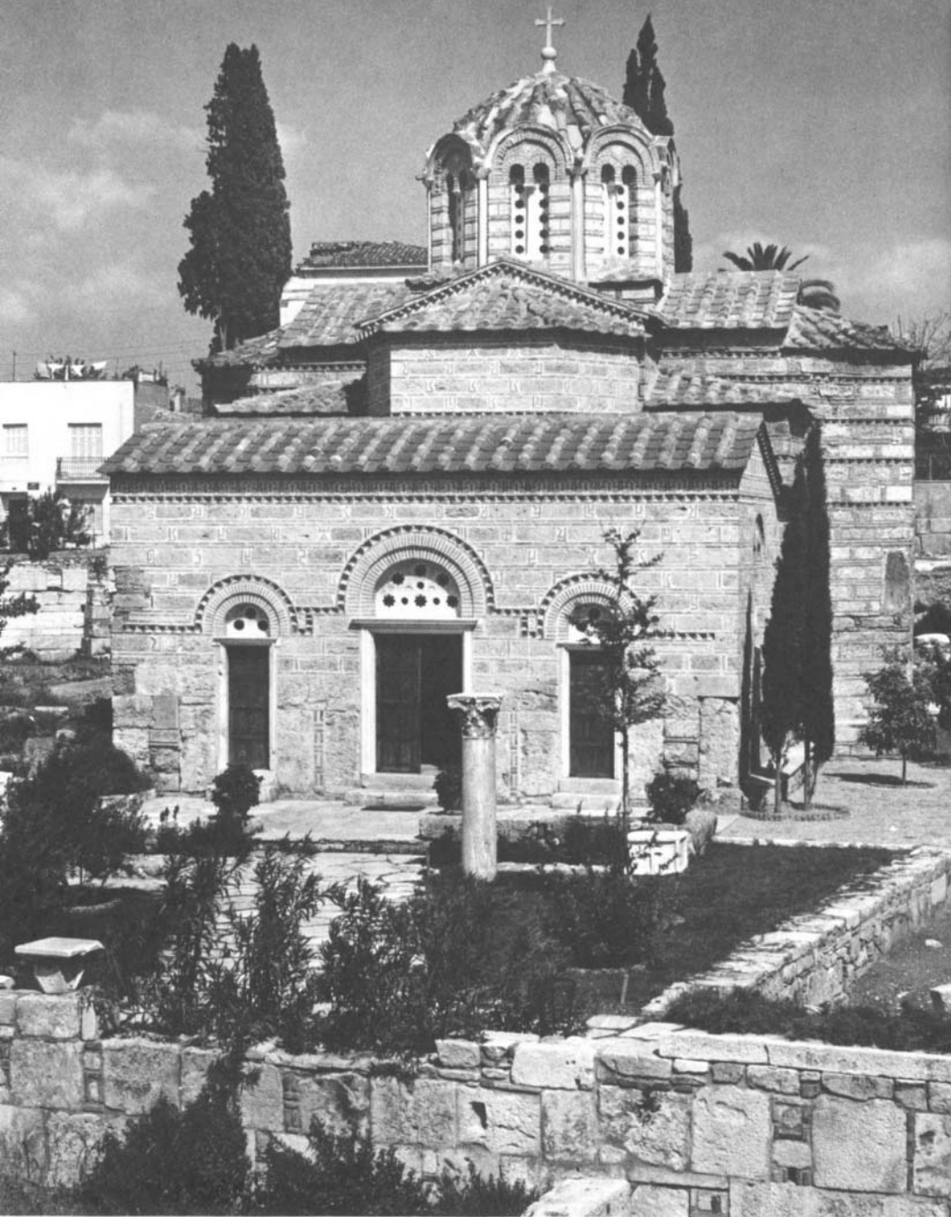
58. The Holy Apostles. Exterior after Restoration.
