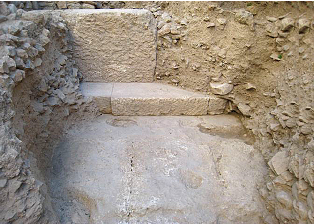
Fig. 2: Back wall of the Painted Stoa from inside, toichobate and orthostate at rear, earlier foundation in foreground.
