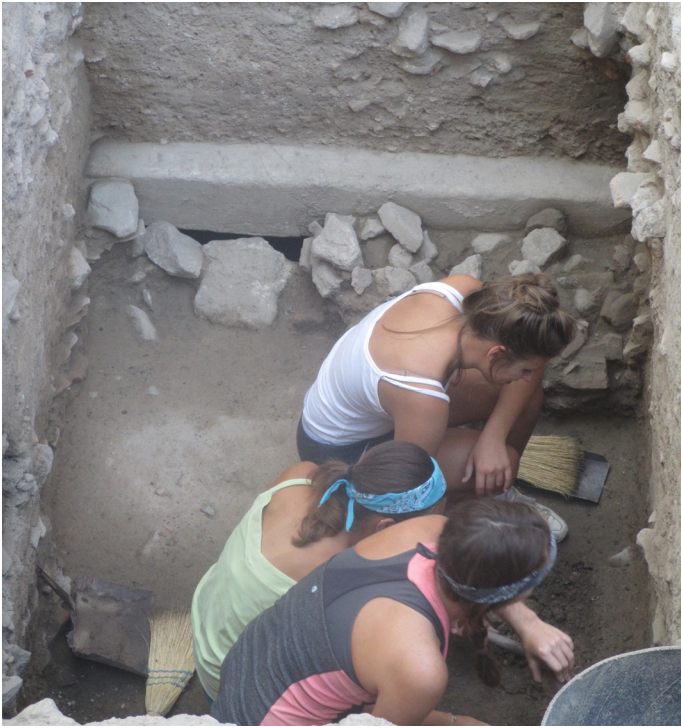
Fig. 6. Larger trial trench with the edge of the cover slab over the river.
